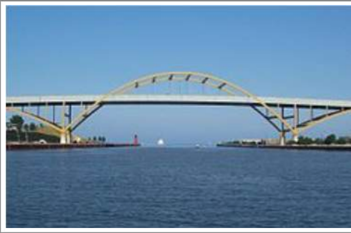
PHOTO: A view of the Hoan Bridge over the Milwaukee Harbor
